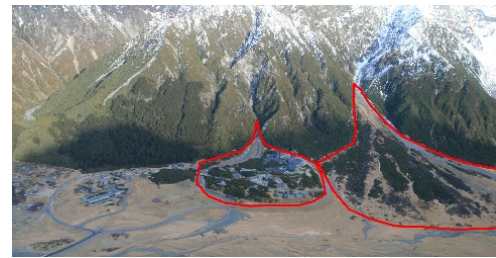
Mt Cook Village – built on debris flow fans
